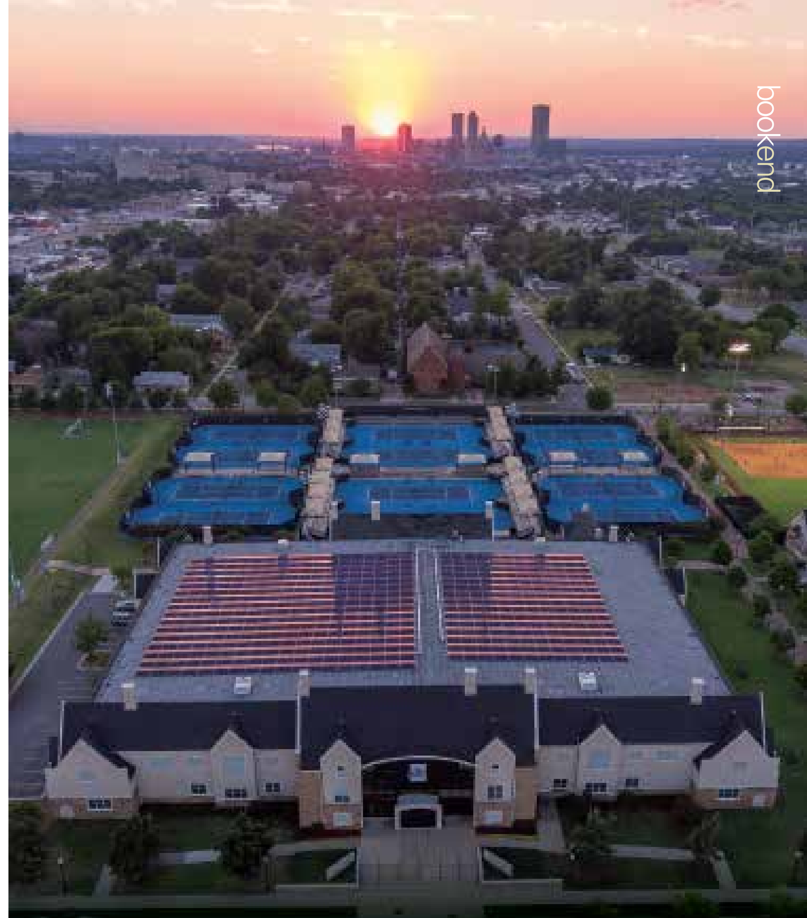
TU's Case Tennis Center is being powered by solar energy in partnership with Public Service Co. of Oklahoma. On Sept. 28, 2016, TU and PSO officials announced completion of the four-month project, one of the state's largest rooftop solar installations. The implementation of solar power supports TU's ongoing efforts to promote a campus culture focused on increasing sustainability.
